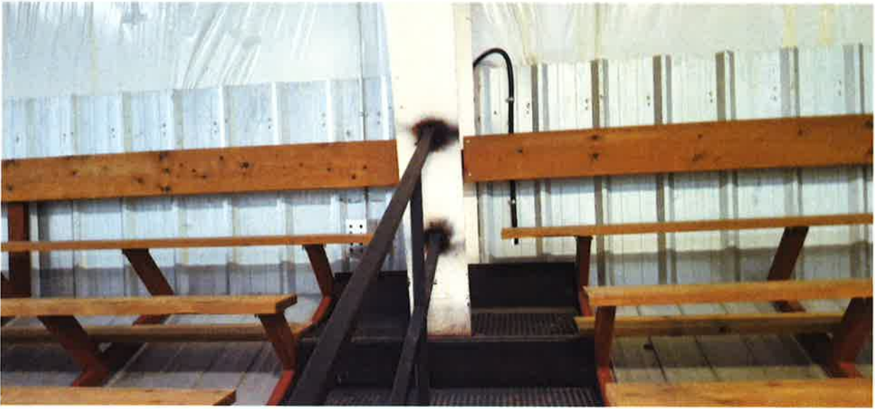
Photo 10: Handrails welded to building frame.
