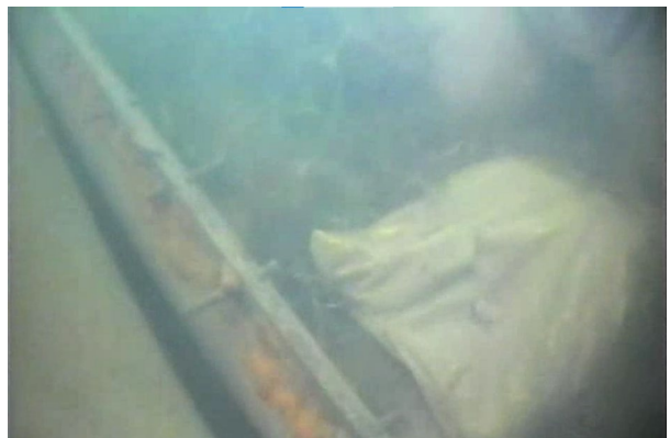
Photograph 6: Chlorine line conduit repair
