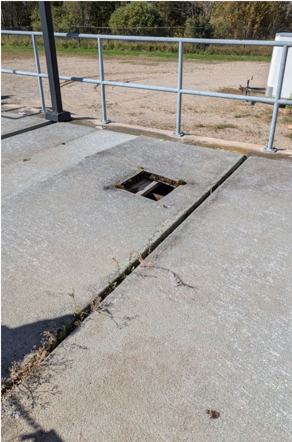
Photograph 8.3: Insulated Secondary Clarifier Covers
