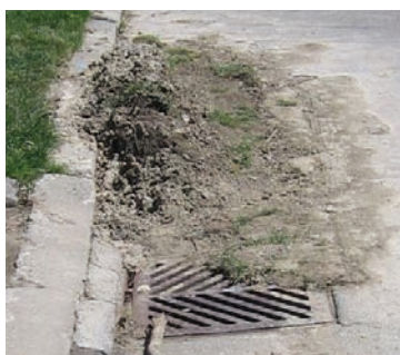
Storm sewer grates that are free of debris are better able to handle stormwater flows and can reduce overland flooding.
